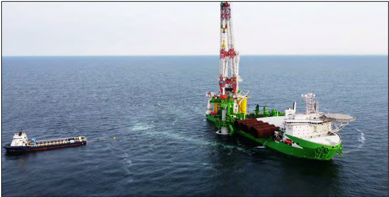
Figure 1. The Orion, drone view, in Vineyard Wind lease area. Photo by DEME [1], shows Orion (right) at stationary position with hammer on starboard side, monopile sections in laydown amidships. Bubble curtain support vessel at left.
